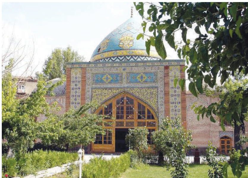
A part of the Blue Mosque after restoration. The year 2006.
